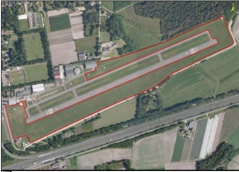
Urban Vegetated Areas (Airport Area)
